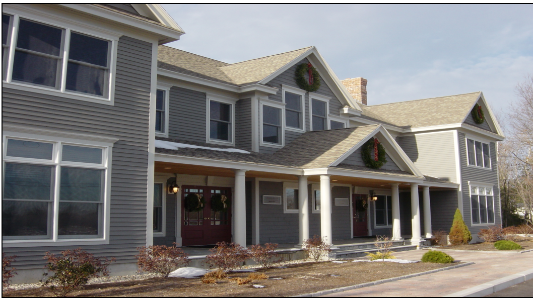
Buildings with multiple uses or tenants shall be designed with a complex massing that includes varying roof lines, projections/recesses, or smaller additions to a main building.
