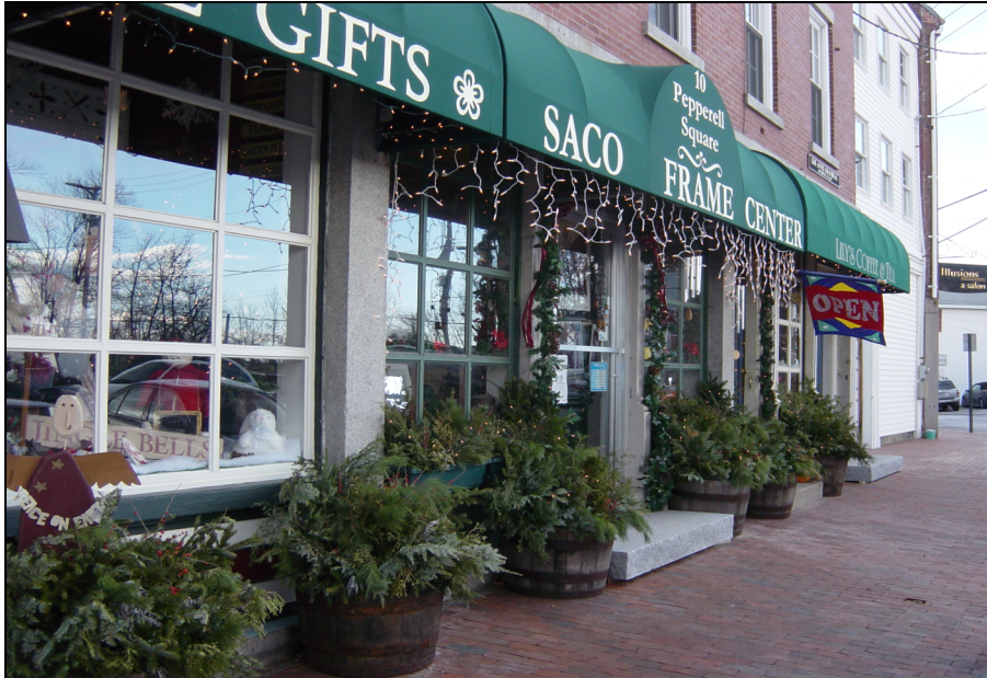
Awnings (temporary and movable) and canopies (permanent) are encouraged in order to visually integrate a series of buildings through compatible or coordinated placement and design.
