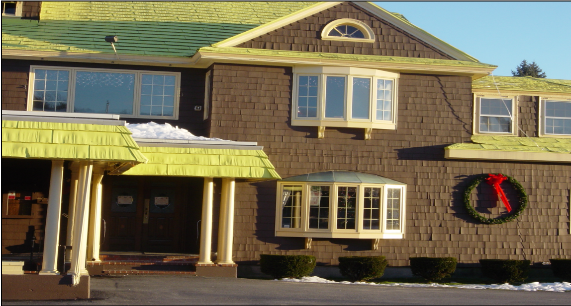
The gables, bay windows and shingle siding contribute to the traditional New England appearance of this building.
